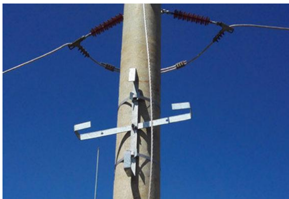
Figure 7 (b) FOC Storage Kit Assembly with mounting straps
